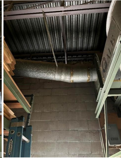
Ductwork piping to transport sawdust
